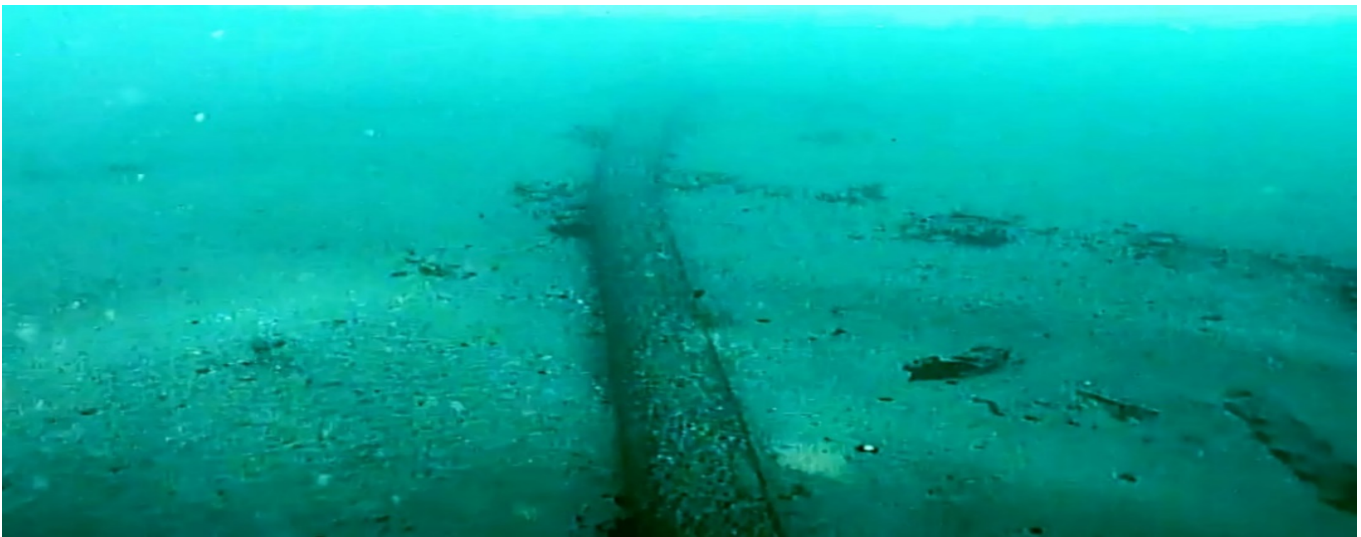
Figure 5 - USCG released image of the displaced Amplify Energy pipeline, 05 th October 2021
